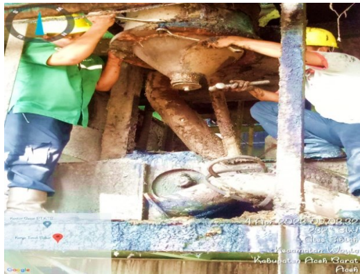
Gambar 6. Proses penggantian cone kernel hydrocyclone
